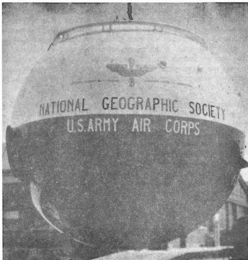
FIGURE 47. Stratosphere Gondola; Magnesium-alloy Sheet
